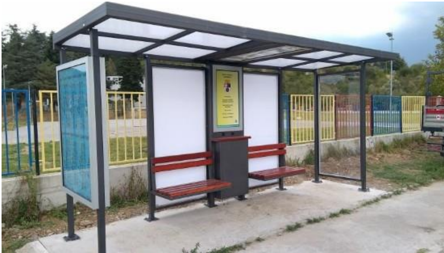
Figure 2. Smart bus stop in municipality Voždovac, Belgrade [6]
