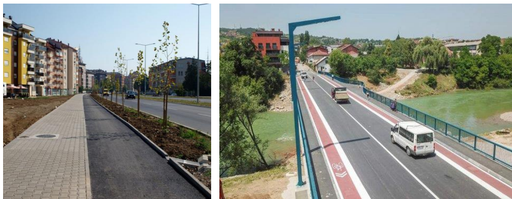
Figure 7. Construction of cycling infrastructure
