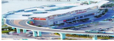
Figure 5. Elevated route for bus rapid transport
