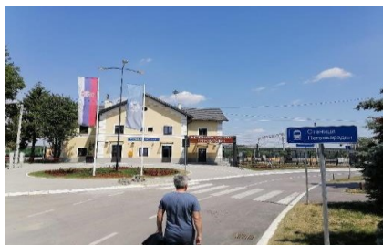
Figure 13. Station building main entrance (source: photo author)
