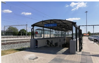
Figure 15. Platform with stairs to underpass (source: photo author)
