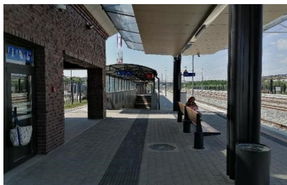
Figure 10. Platform with stairs to underpass (source: photo author)
