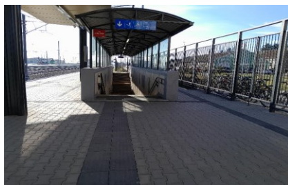
Figure 2. Platform with stairs to underpass (source: photo author)
