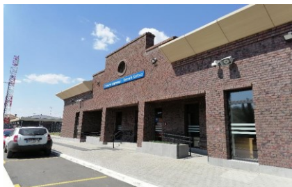
Figure 9. Station building main entrance and parking space (source: photo author)
