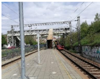
Figure 5. Access to the platform and platform
