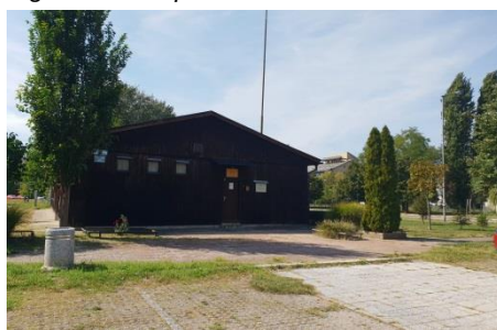
Figure 4. Cultural station under construction, Novo Naselje
