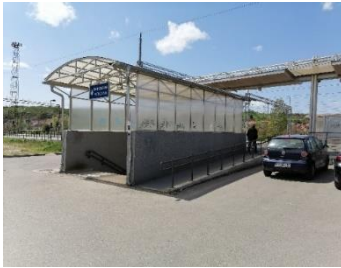
Figure 8. Access to the underpass, platform and parking lot
