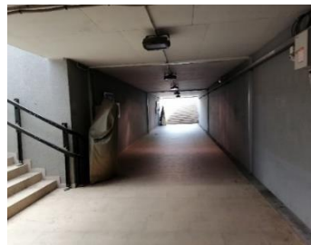
Figure 11. Access to the platform from the underpass with movable platforms
