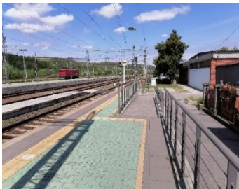
Figure 10. Access to the platform
