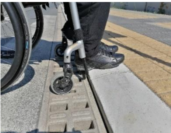
Figure 13. Curb on the pedestrian road next to the station
