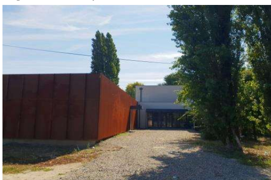
Figure 3. Cultural station under construction, Klisa
