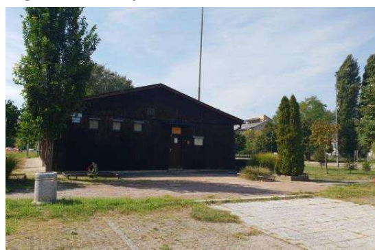
Figure 4. Cultural station under construction, Novo Naselje
