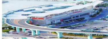
Figure 5. Elevated route for bus rapid transport
