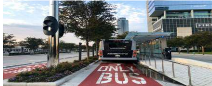
Figure 2. Physically separated route for bus rapid transport
