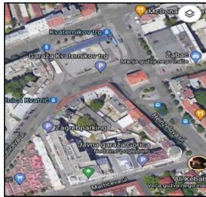
Figure 1. Public garages Katernikov trg and Gorica – aerial view [12]
