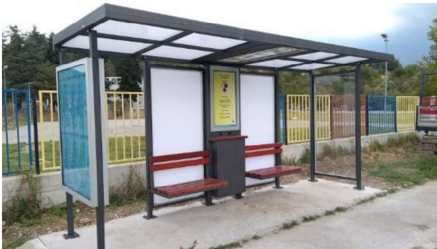
Figure 2. Smart bus stop in municipality Voždovac, Belgrade [6]
