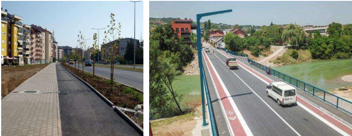
Figure 7. Construction of cycling infrastructure
