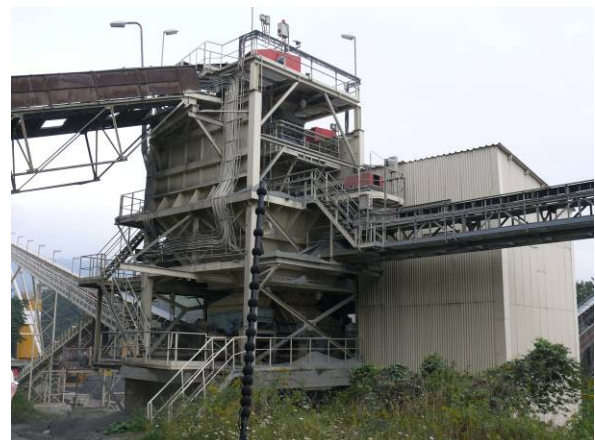
Fig. 10. Installed Acoustic Camera by crushing plant.
