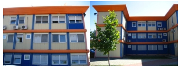
Fig. 2 b. Intermodal steel building units in Novi Sad, Serbia for office purposes
